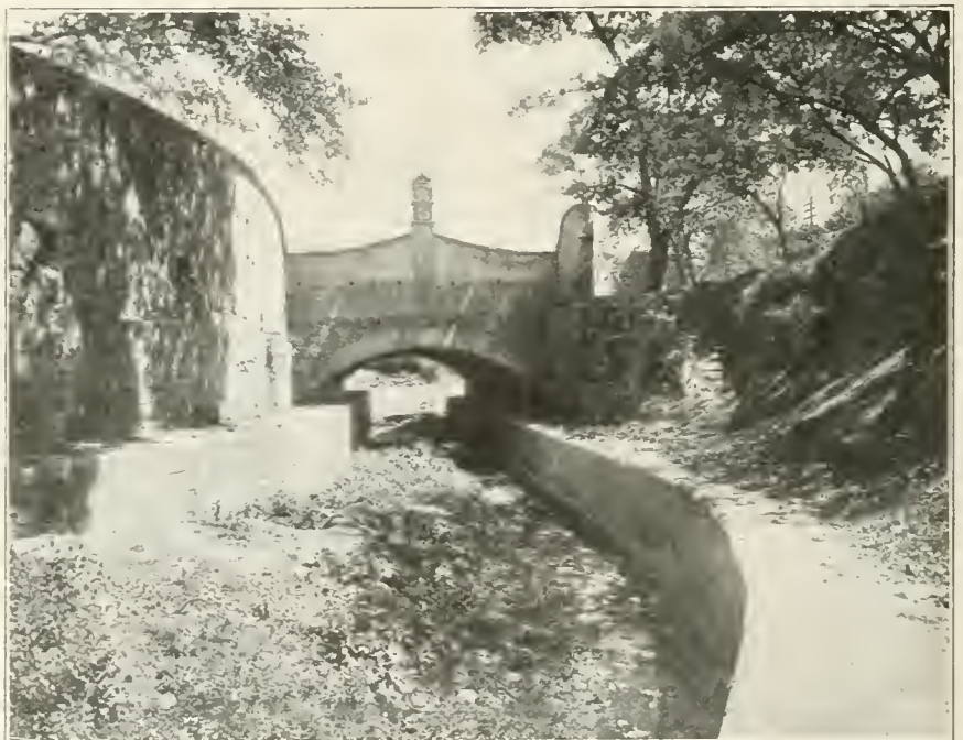
Marino Bridge, showing parallel sewers. The sewers, laid in pairs in the beds of the quebradoes, are carried to the trunk line which parallels the Rio Guaire, into which the sewer eventually empties.
